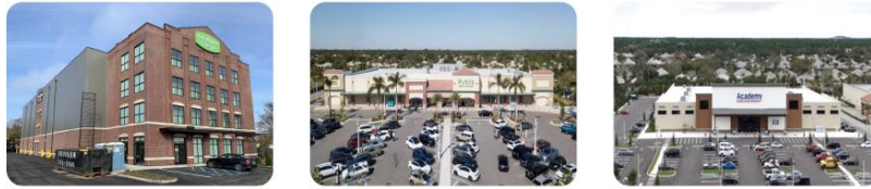
Figure 14: Asset enhancement works
